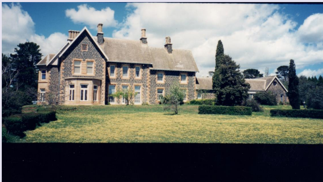
Bishopthorpe – Conference Centre Goulburn NSW
